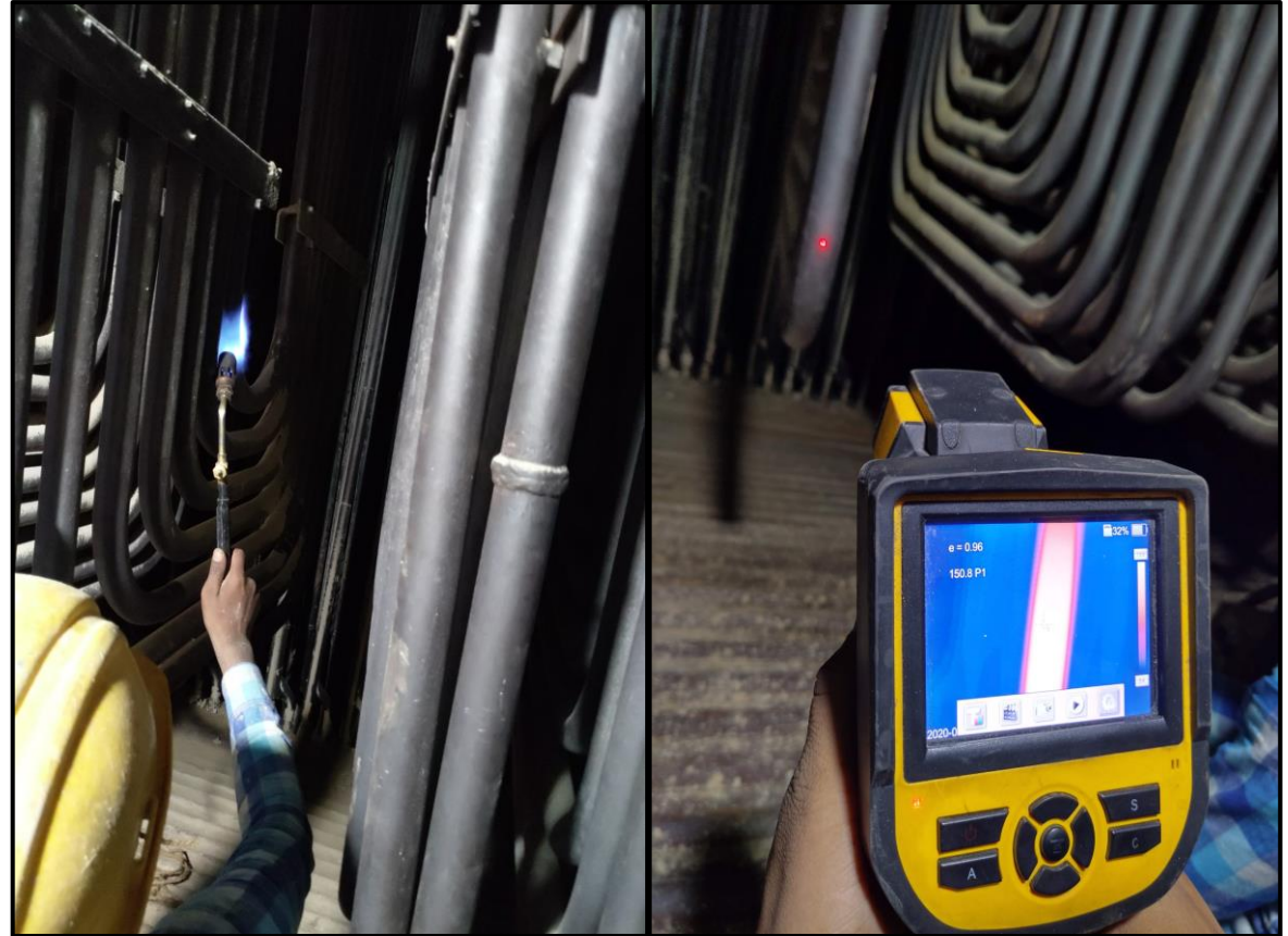
(b) Heating bends by flame torch
