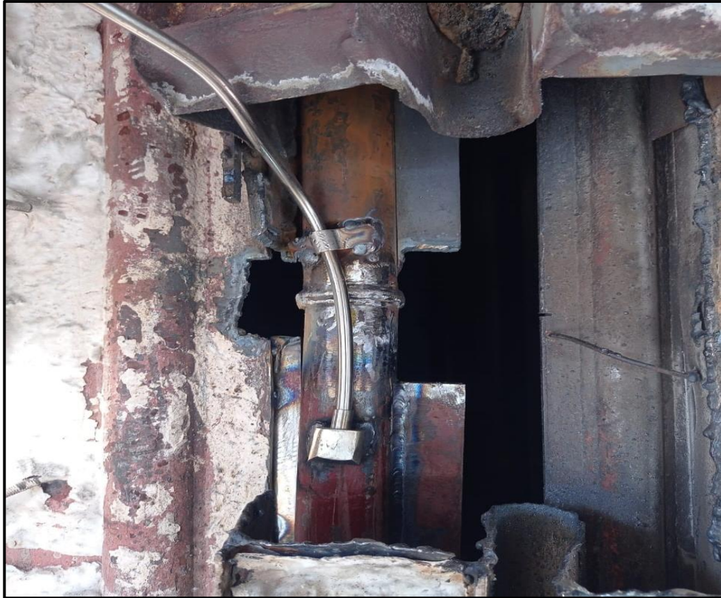
(a) Installing & Monitoring MTMs
