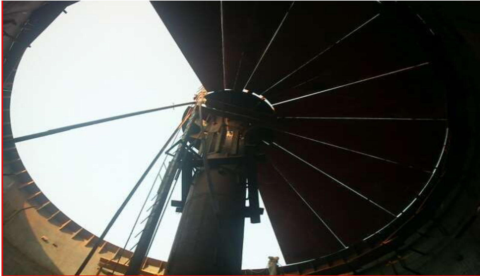
Anaerobic Reactor Roof
