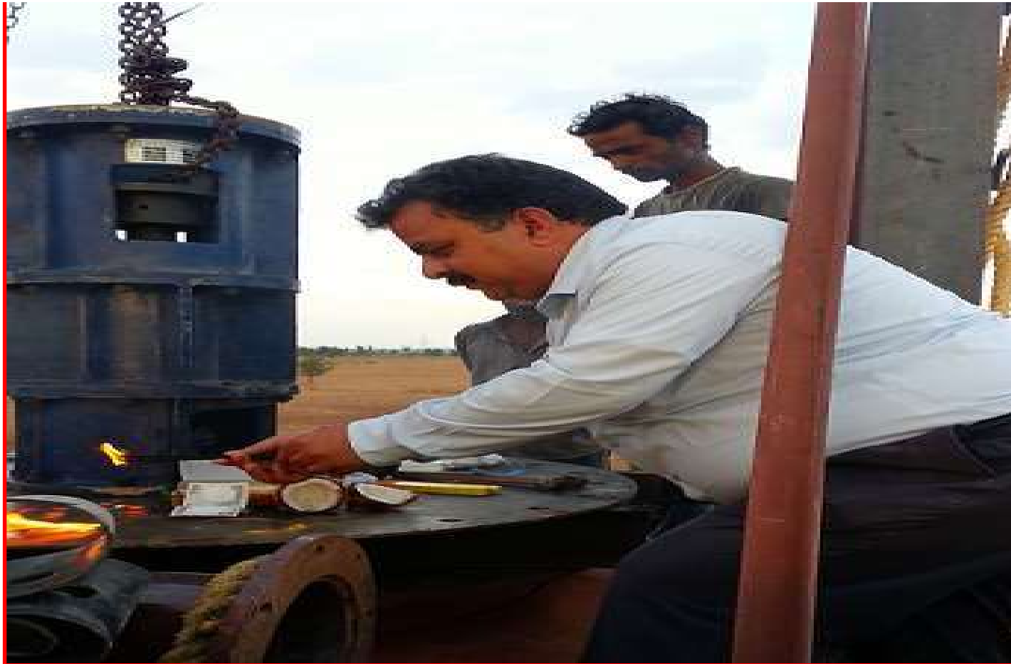
Mounting of Central Agitator On Reactor Roof
