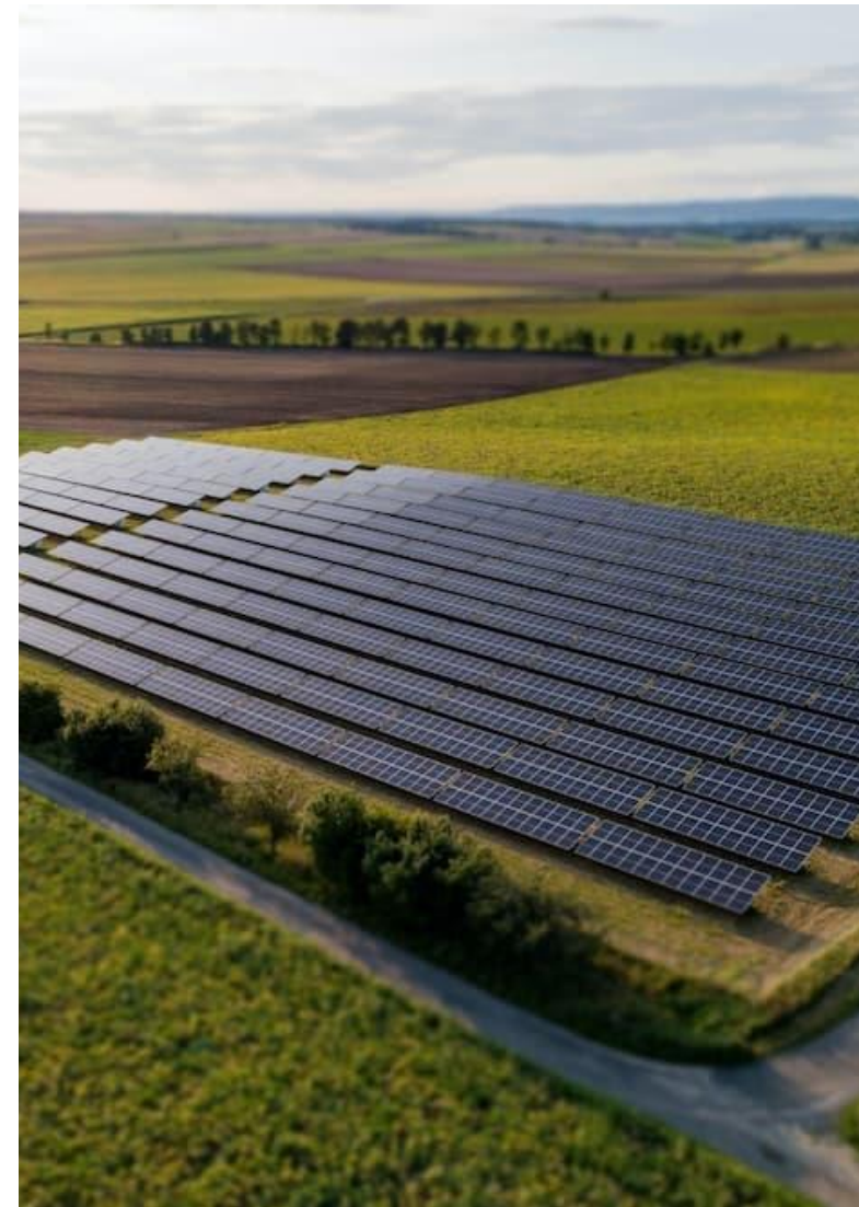
Rooftop & Solar Farm
