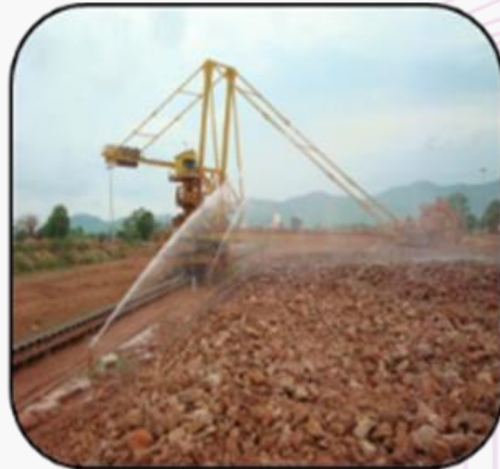
Water sprinklers at bauxite handling
