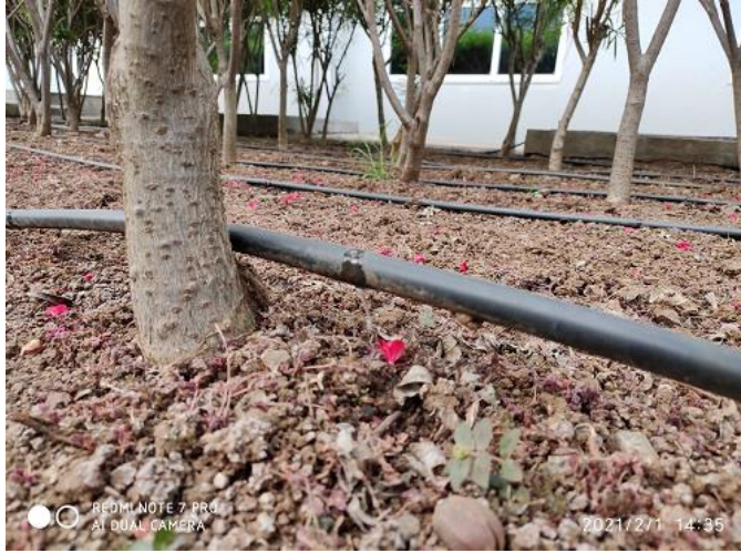
Drip irrigation System
