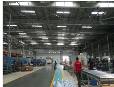
Day lights Roof sheets
