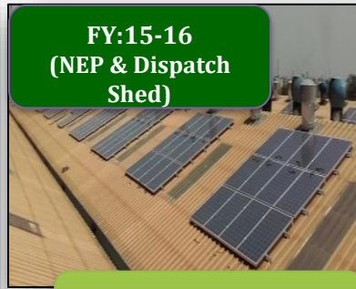
250 KWp Roof-top Solar PV System
