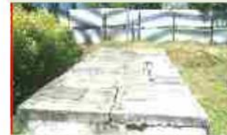
Rain water Pit
