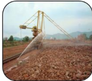
Water sprinklers at bauxite handling
