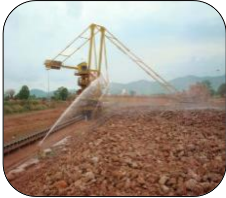
Water sprinklers at bauxite handling
