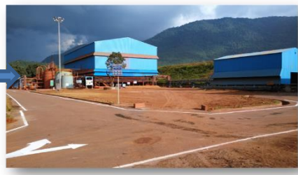
Red mud Filtration unit
