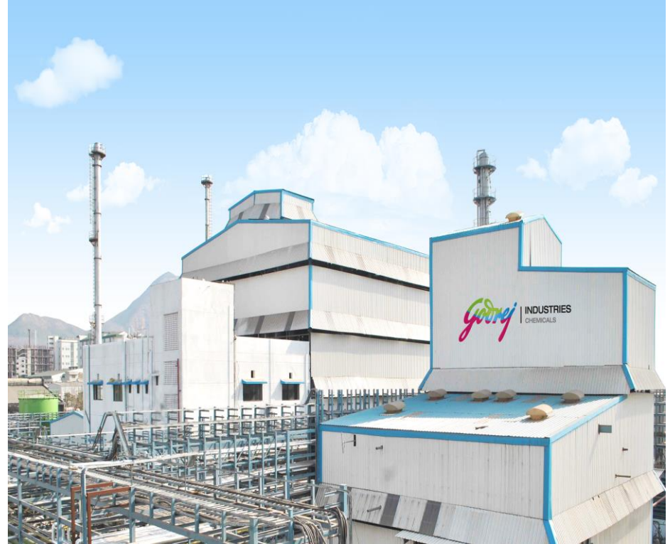
Manufacturing Plant in Maharashtra
