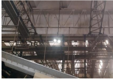
Lifelines on trusses in PMD
