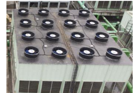
BLDC fans for cooling towers
