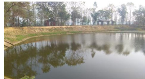
Building Sustainable Infra in Saharanpur
