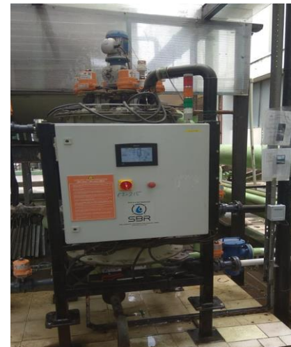
Scale and bio removal for Cooling tower Net Impact-1000 KL
