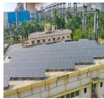
Roof of Control Room
