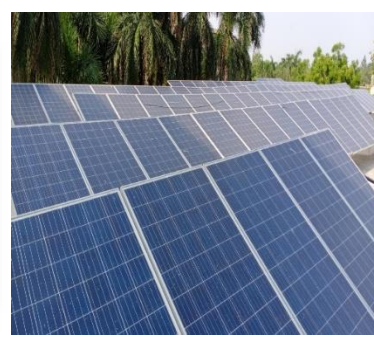
Roof of Central Canteen
